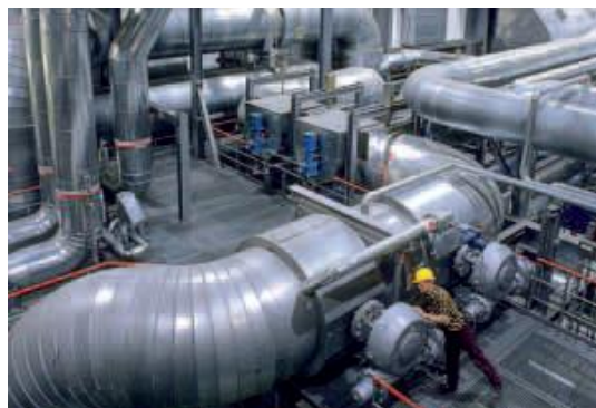
Fig. 8 Nanotech coating of oil pipes [27].
